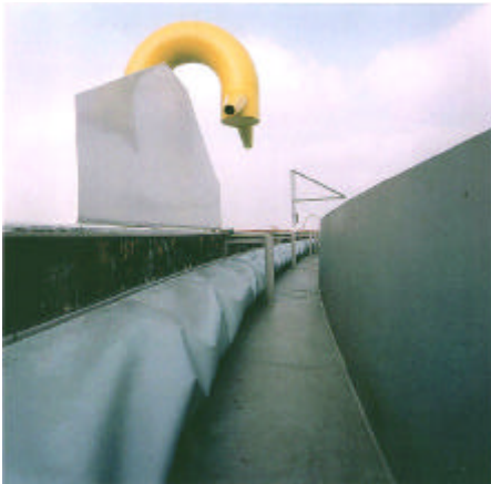
Secondary SealMaster from above deck
