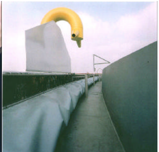
Secondary SealMaster from above deck
